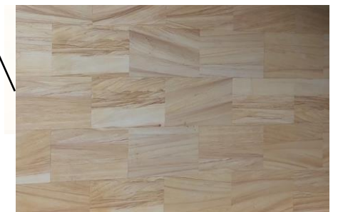
Stone Facing – Natural Sandstone stretcher pattern
